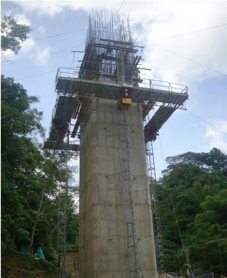
Working Platform for a bridge building (Colombia)
