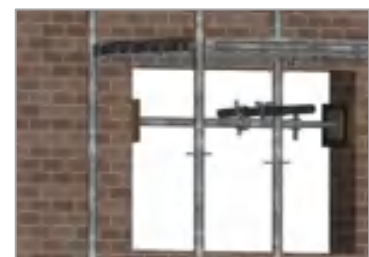
Shoring up windows
